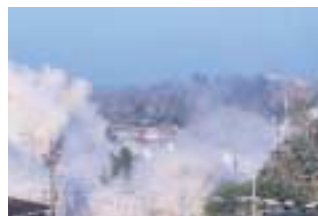
Seven-story Voorhies Dorm was reduced to rubble on Feb. 1.
