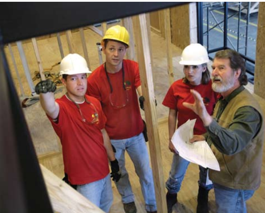
Professor Emeritus Eddie Cazayoux and architecture students make sure everything goes according to plan; he has been involved with the BeauSoleil project since its inception. Shown, from left, are: Christopher Leger, Jeremy Credeur, Gretchen Lacombe-Vanicor and Cazayoux.
