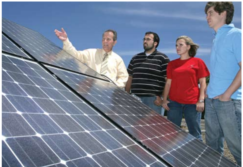
To test their design, team members installed solar panels on the roof of Madison Hall on the UL Lafayette campus. The panels feed energy back into the university's power system. Shown, from left, are: Dr. Robert Henry, a UL Lafayette engineering professor; engineering student Thomas Bosch; and architecture students Gretchen Lacombe-Vanikor and Scott Chappuis.
